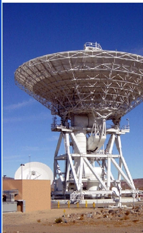
Figure 3: DSS 25, a 34-m beam-waveguide antenna, shown here in the stowed position. DSS 25 is one antenna in the NASA/JPL Goldstone Deep Space Communications Complex near Barstow, CA, U.S.A. It has special instrumentation (Ka-band uplink and advanced media calibration capability).
